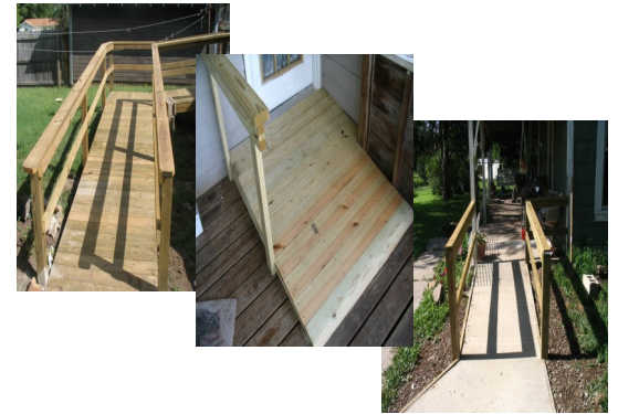
Long ramp, short ramp and connection ramp
