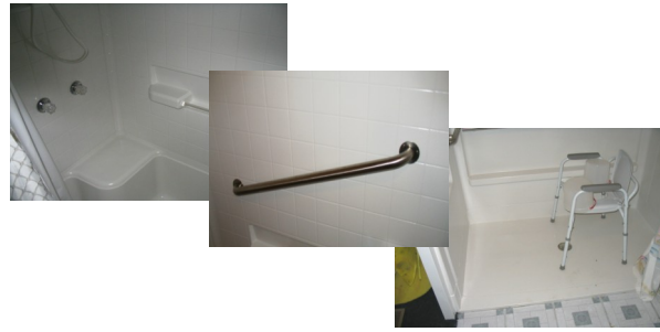
Accessible Shower Unit with built-in chair, with removable chair, grab bar installation.
